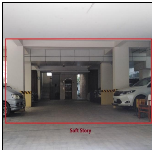
Photograph 3: Appearance of Soft Story Photograph 4: Pounding between Adjacent Building
