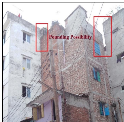
Photograph 3: Appearance of Soft Story Photograph 4: Pounding between Adjacent Building
